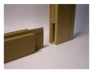
Mortice and tenon joint
